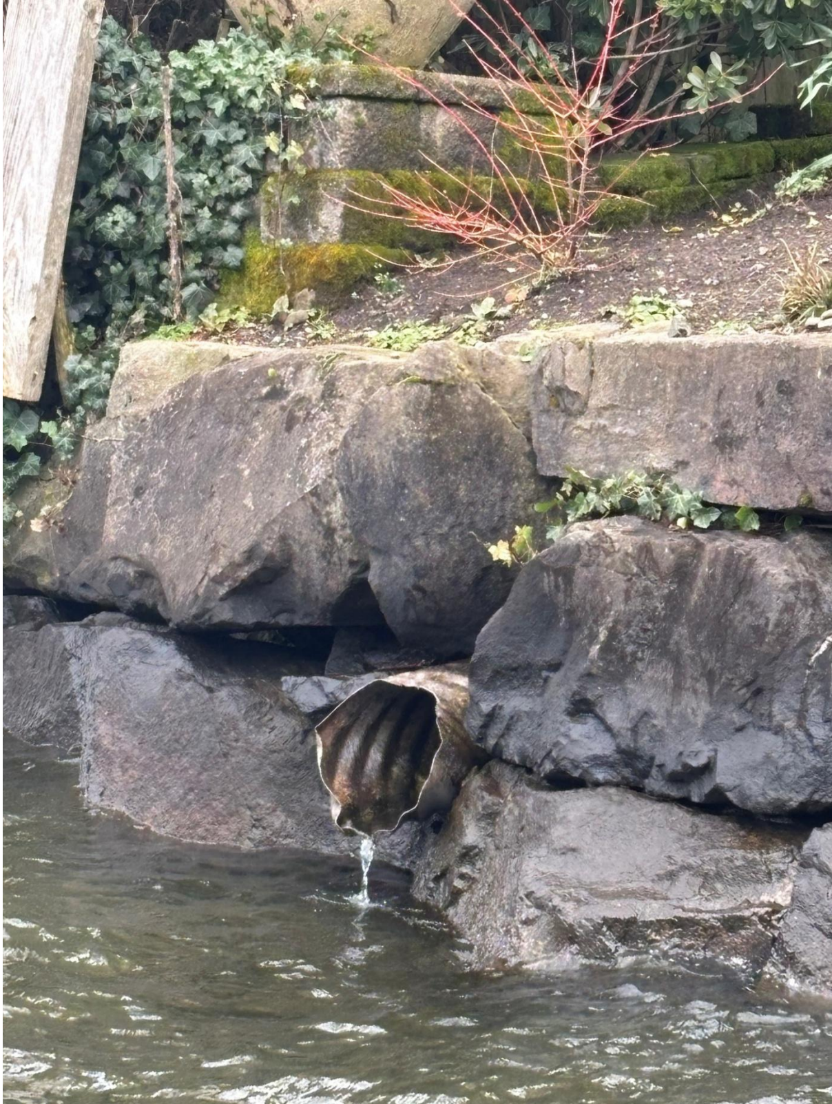
View of storm drain outflow in Lake Washington
